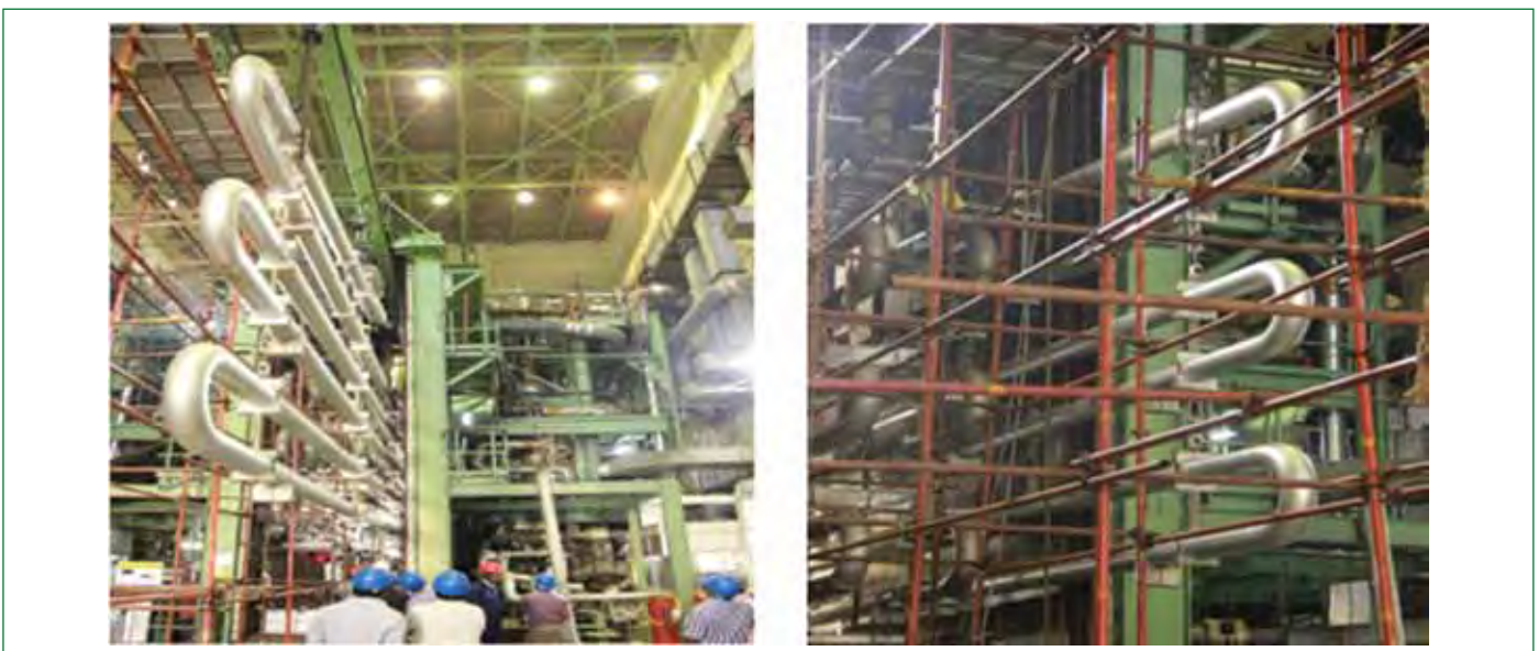
Figure 3: Steam generator module installation
