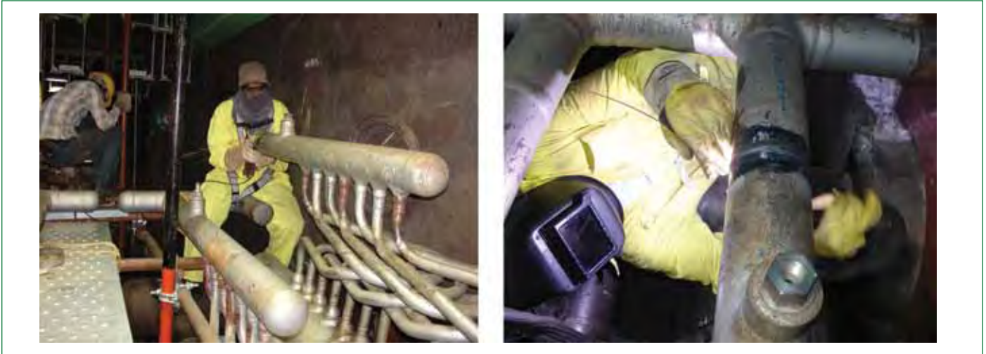
Figure 4: Joint fit up and welding with system headers
