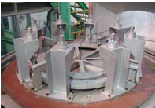
Fig. 1 Back-up seal test rig inside heater shell
