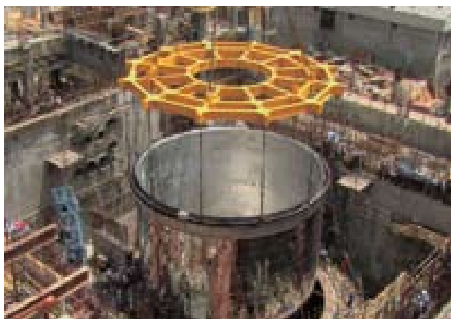
Fig. 2 Erection of safety vessel
