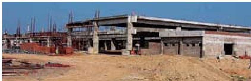
Fig. 2 Work on stores building in progress at FRFCF site
