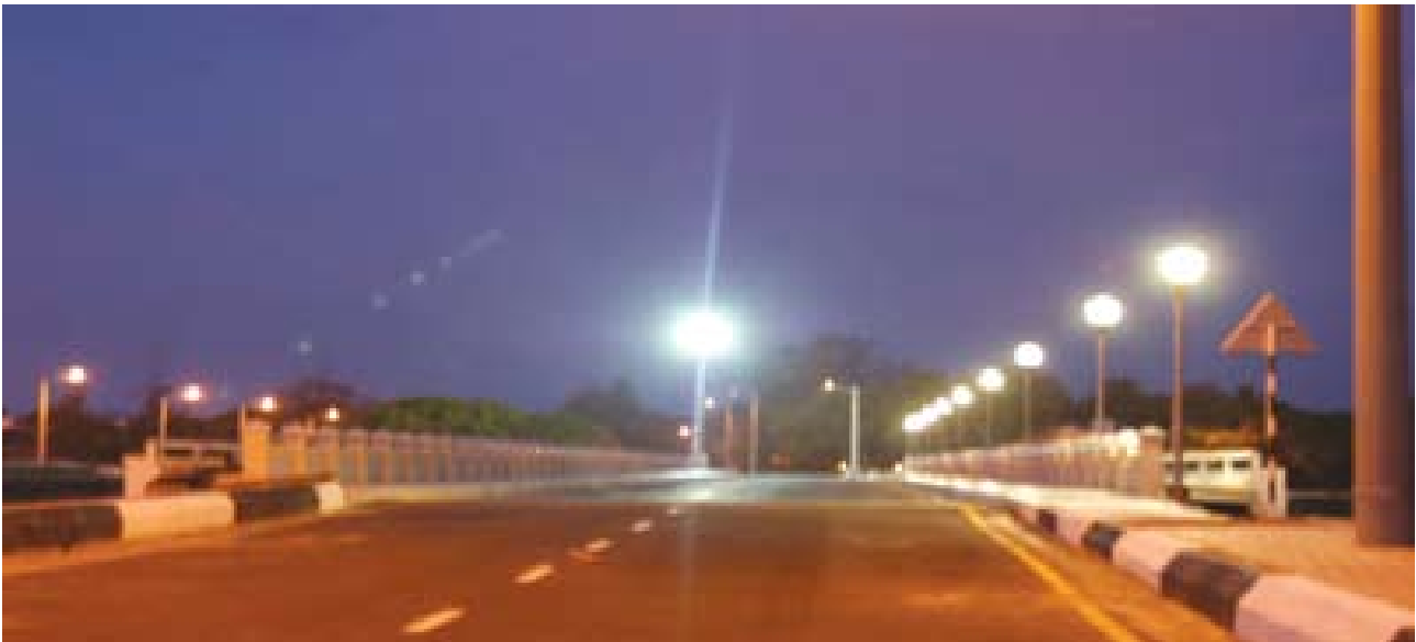
Fig. 4 View of the bridge from Sadras side
