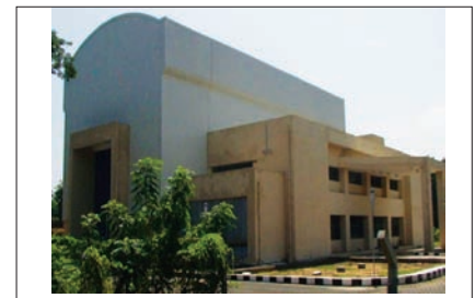
Fig. 1 Structural dynamics laboratory
