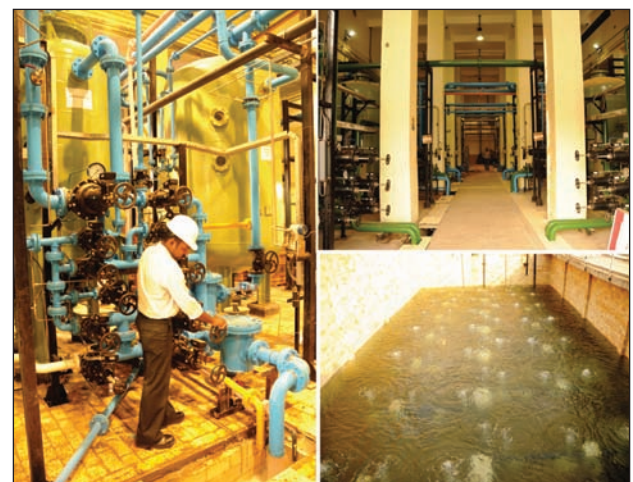
Fig. 7 Commissioning of de-mineralized water plant
