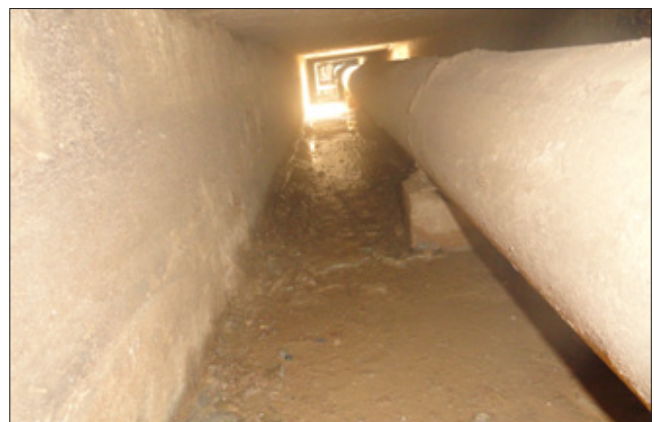
Fig. 3 Tunnel before SCC
