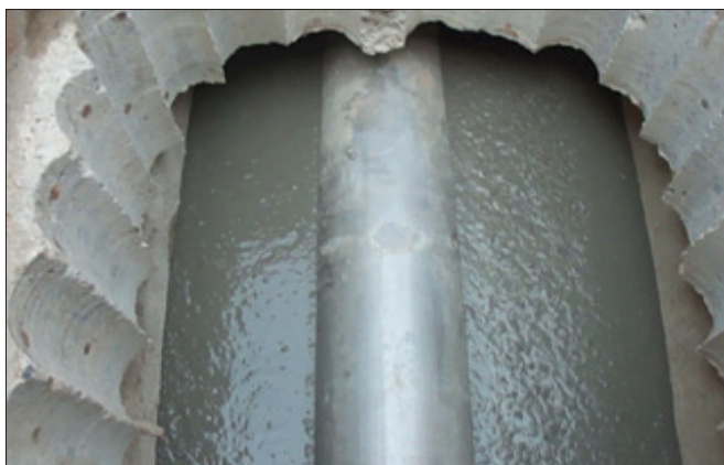
Fig. 2 Pouring of self compacting concrete into the trench
