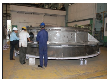
Fig. 2 Box structure (in inverted position) after assembly of top and bottom plates and shells
