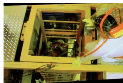
Fig. 2 Repair crew in ventilated suit entering the cell
