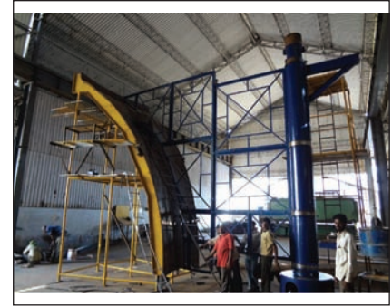
Fig. 6 Profile measurement of inner vessel sector using swing arm arrangement
