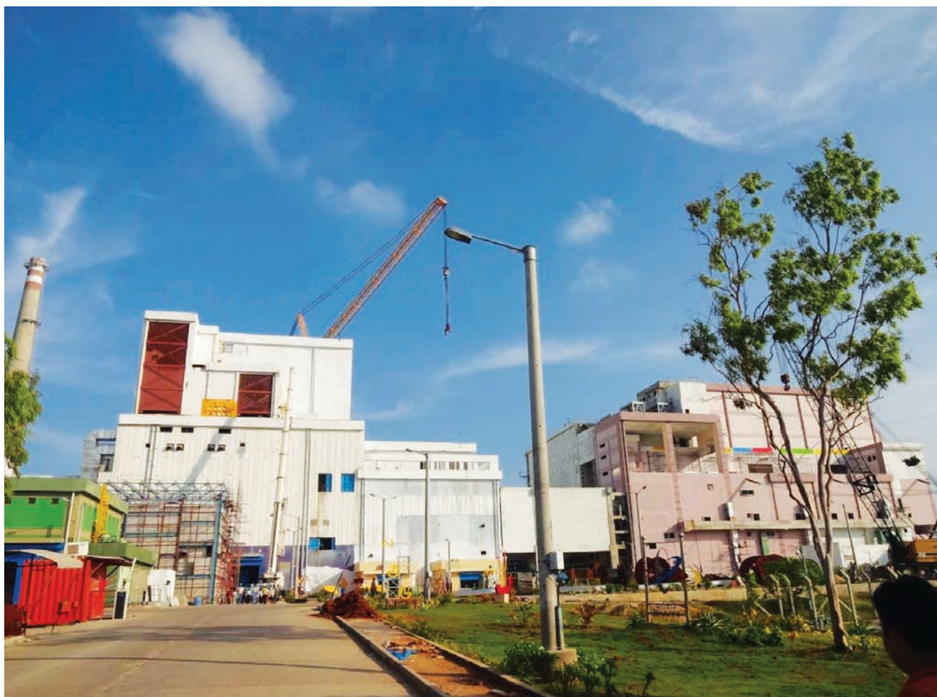
Fig. 1 Overall view of nuclear island connected buildings
