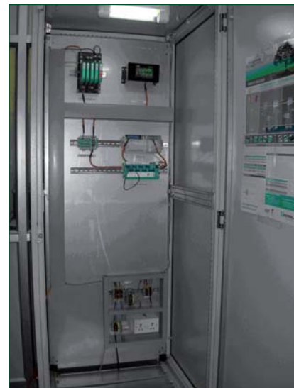
Fig. 3 Laboratory setup of foundation fieldbus for distributed temperature measurement
