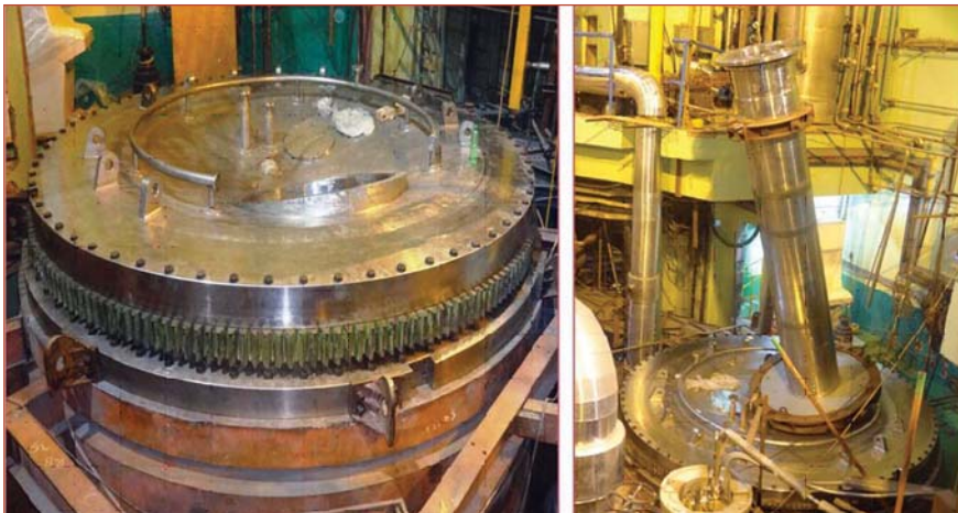
Fig. 1 Erection of inclined fuel transfer machine
