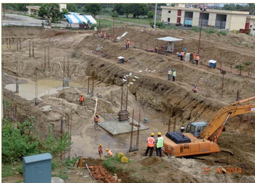
Fig. 2 Backfilling in progress for extension of stores building of FRFCF
