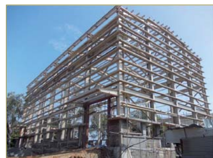
Fig. 2 Photograph of facility building under construction
