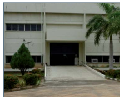
Fig. 2 Truck entry areas provided with ramps
