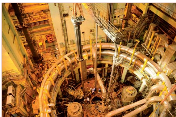
Fig. 2 Transfer arm erection
