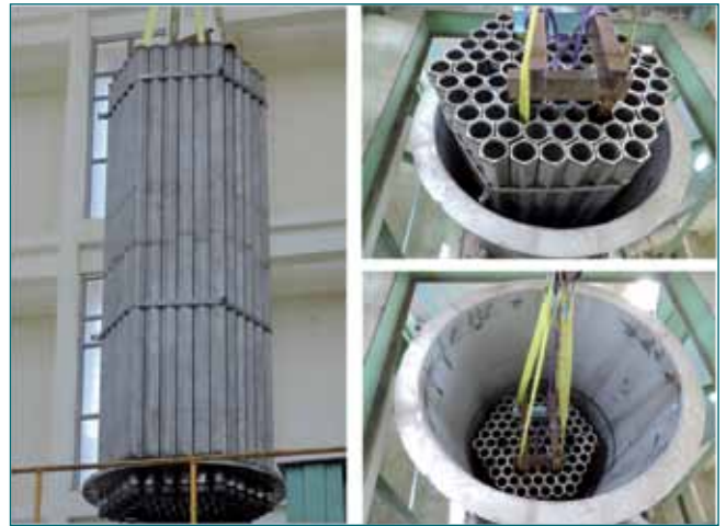
Fig. 2 Erection of core assembly in test vessel
