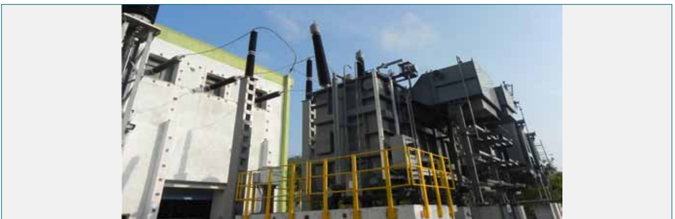
Fig. 1 47 MVA transformer
