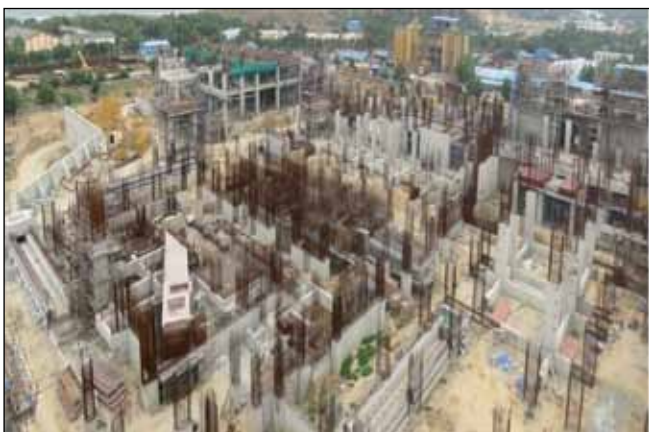
Fig. 1 Waste management plant
