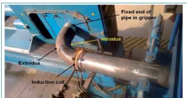
Fig. 4 Final primary pipe 110° bend
