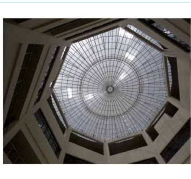
Fig. 2 Internal view of the skylight
