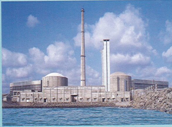
Madras Atomic Power Station (MAPS)
