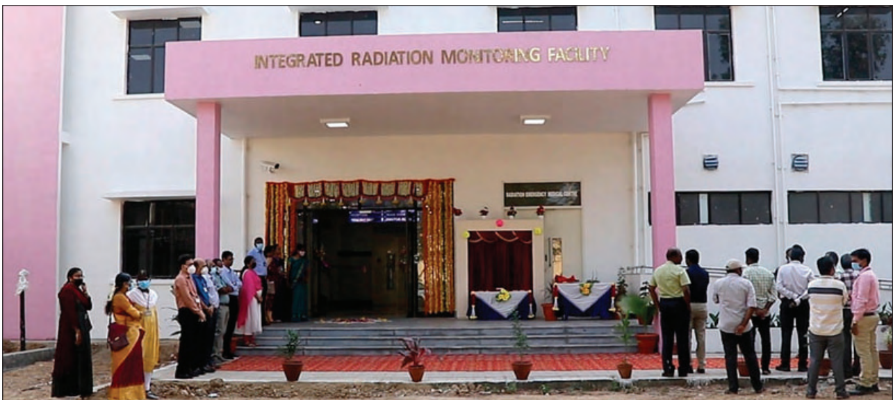
Integrated Radiation Monitoring Facility building at Anupuram
