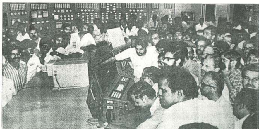
Joyous moment - FBTR Control room after the first criticality.
