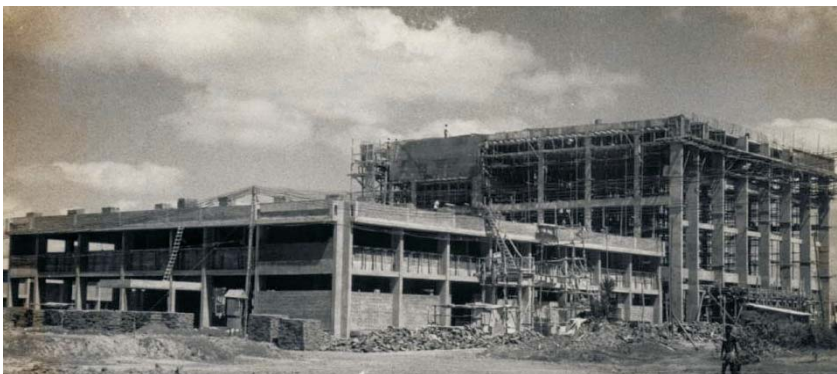
Reprocessing Development Laboratory construction in 1974
