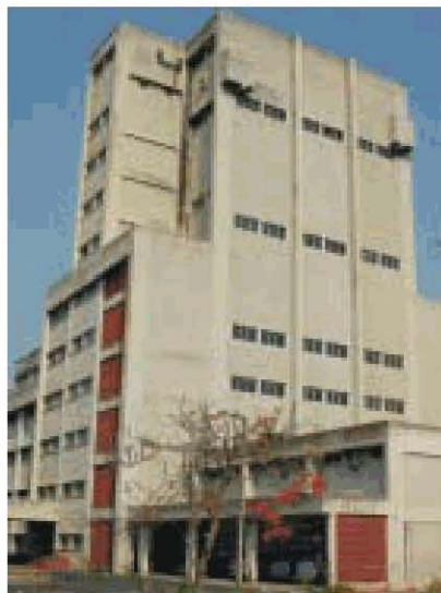
HALL-3 building of FRTG
