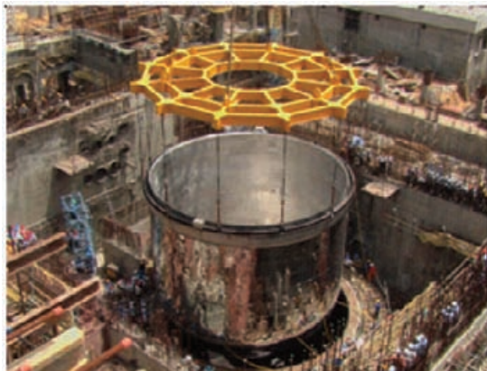
Figure 7: Successful erection of safety vessel on the inner wall of reactor vault in June 2008
