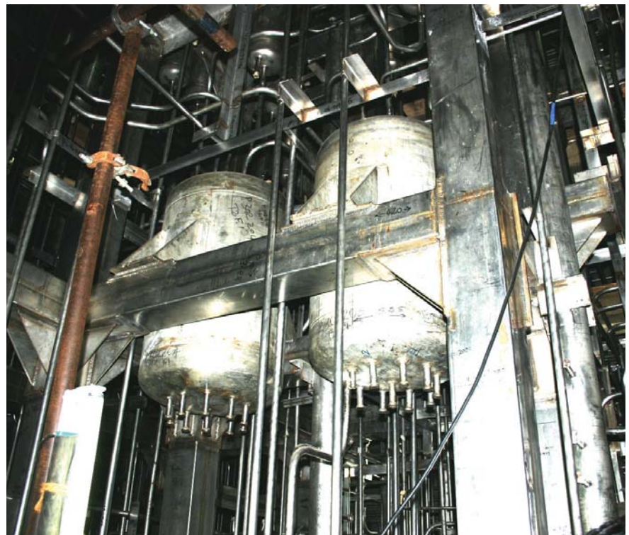
Fig. 1. Equipment and piping erection in the DFRP cell
