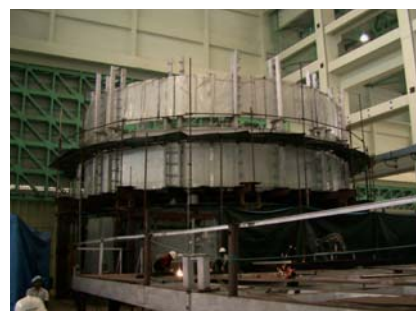
Fig. 2. Safety vessel fabrication
