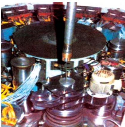
Fig. 2. In-situ cutting of guide tube on the Reactor (1988)
