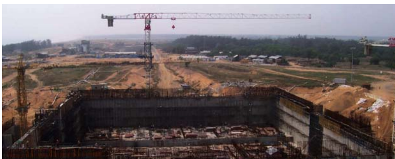
Fig. 1. Construction of PFBR
