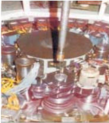
Fig.2 In-situ Cutting of Guide Tube on the Reactor used in 1988
