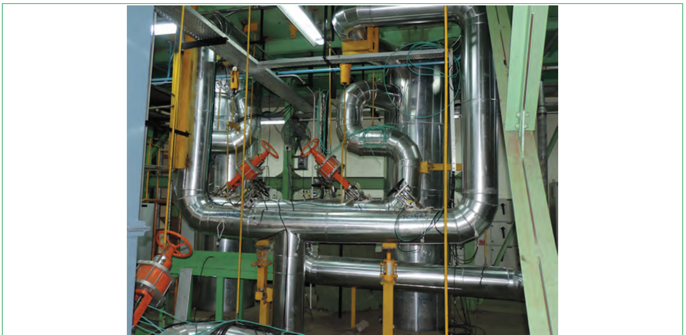
Figure 2: Piping of sodium facility for component testing
