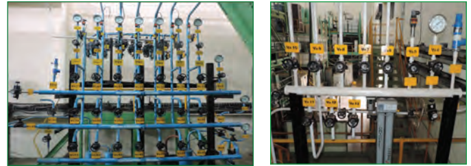
Figure 1: (a) Argon Header of sodium facility for component testing and (b) Compressed air system header of SFCT
