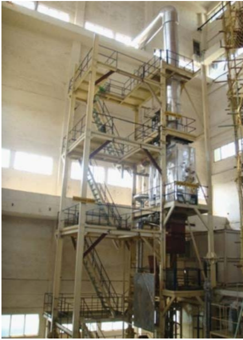
Figure 6: SADHANA Loop with Chimney
