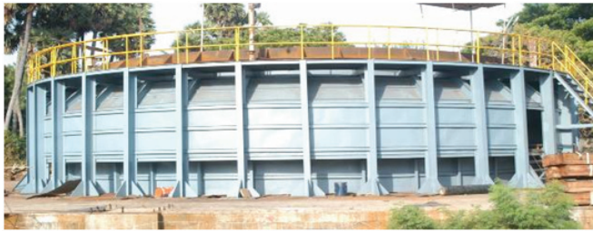
Figure 5: Mockup trials for the successful erection of safety vessel
