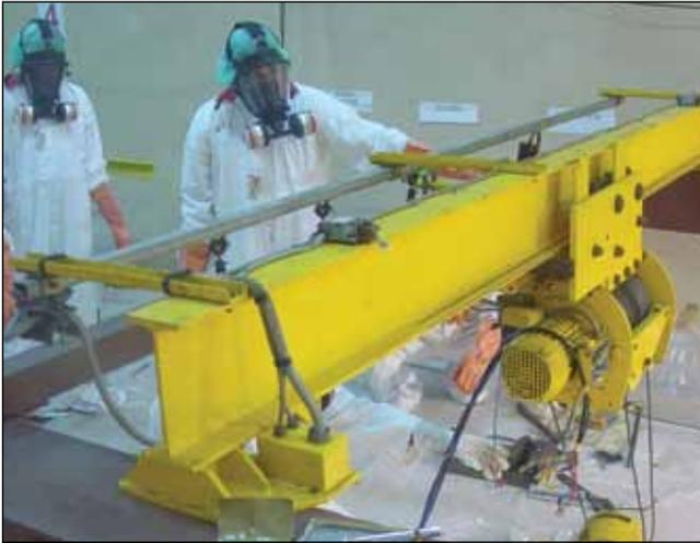
**Fig. 1** Photograph showing personnel engaged in the repair of in-cell crane
