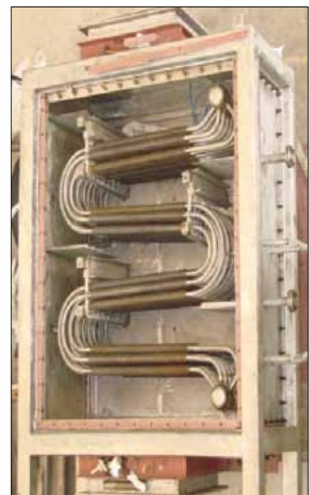
Fig. 2 Air heat exchanger in the side plate opened condition
