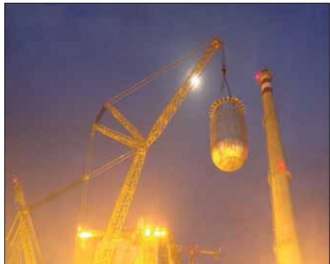
**Fig. 2** Erection of main vessel of PFBR
