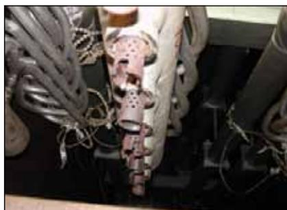
**Fig. 2** Flared ends of water tubes
