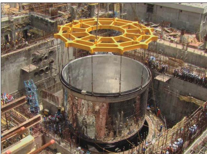
Fig. 1 Safety vessel erection inside reactor vault
