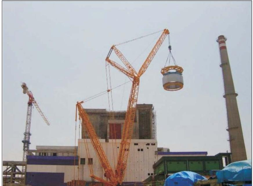
**Fig. 1** Erection of thermal baffle
