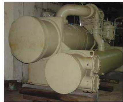
**Fig. 2** 350 TR centrifugal chiller
