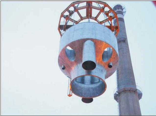
**Fig. 3** Erection of inner vessel
