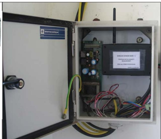
Fig. 2 Wireless sensor network node at SADHANA loop, FRTG
