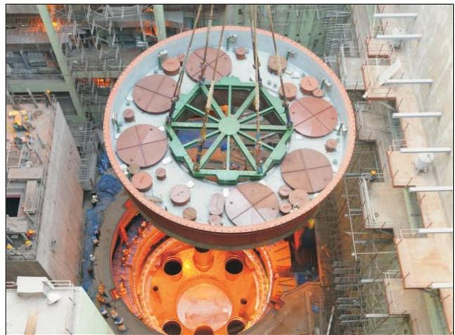
**Fig. 4** Erection of roof slab
