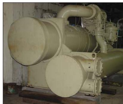
**Fig. 2** 350 TR centrifugal chiller
