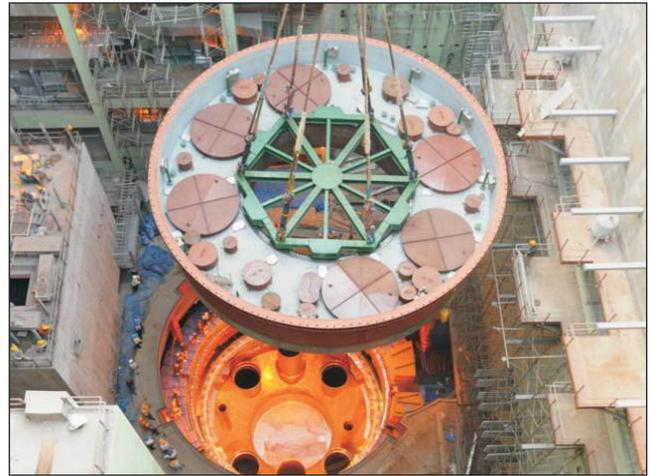
**Fig. 4** Erection of roof slab
