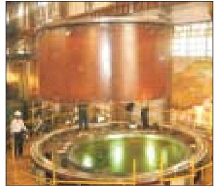
Fig. 7 Assembly of small rotatable plugs within large rotatable plugs
