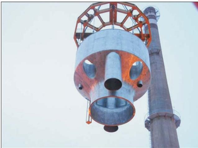
**Fig. 3** Erection of inner vessel
