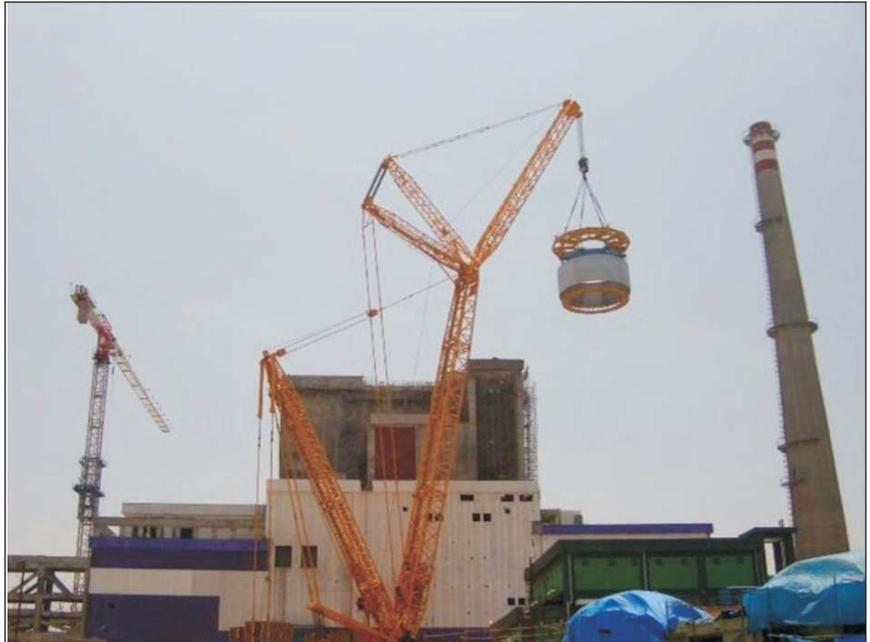
**Fig. 1** Erection of thermal baffle
