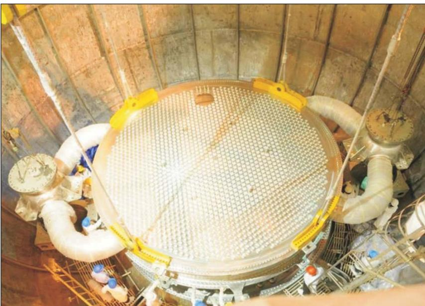
**Fig. 2** Erection of grid plate assembly
