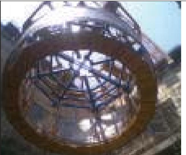
**Fig. 4** Erection of thermal baffle
