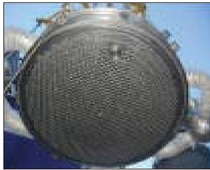
**Fig. 6** Erection of grid plate along with primary pipe
