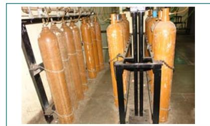
**Fig. 2** Seismic anchoring of gas cylinder banks in the plant
