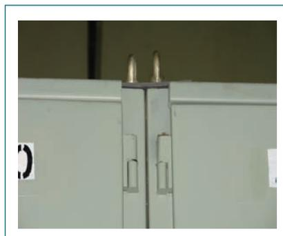
**Fig. 3** Bolting of adjacent panels to avoid seismic interactions
