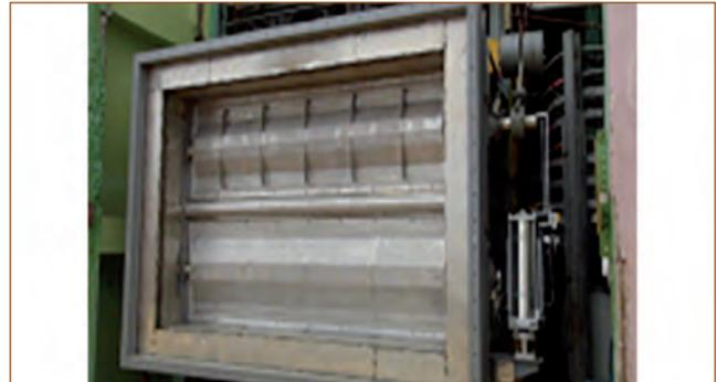
**Fig. 1** Type-A AHX inlet damper-pneumatic
