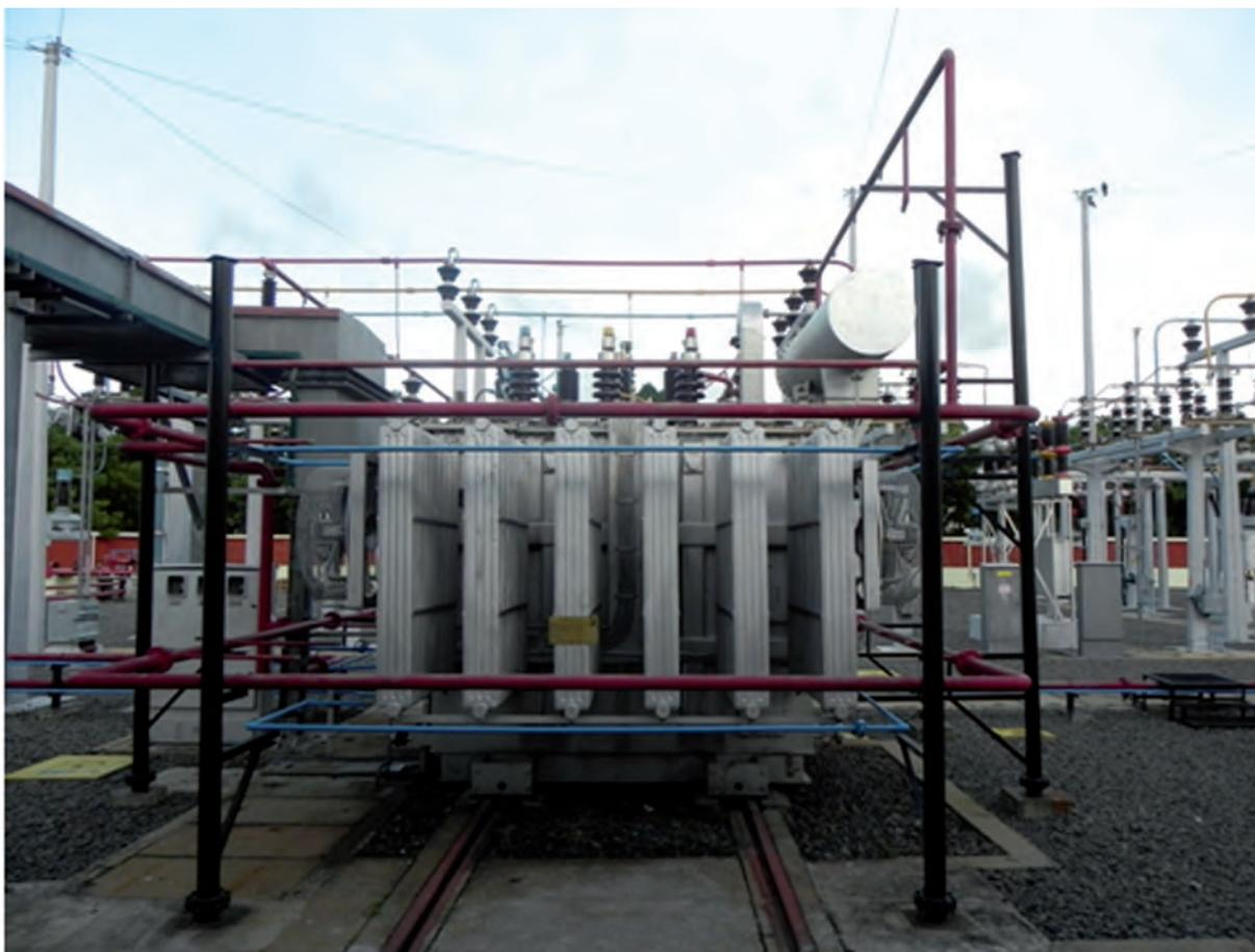
*Fig. 2 33 kV transformer - refurbished*
