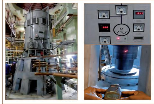
**Fig. 3** Commissioning of secondary sodium pump
