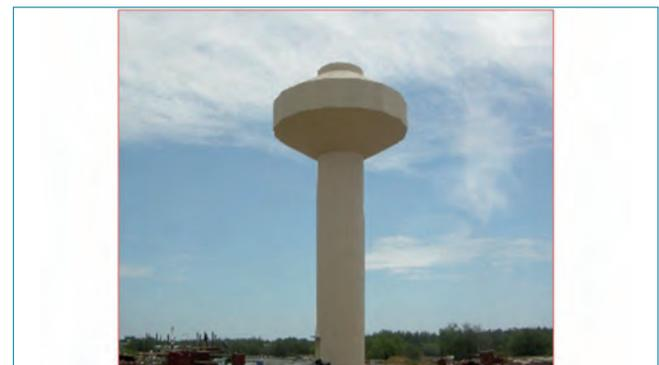
Fig. 12 Picture of completed Intze Tank
