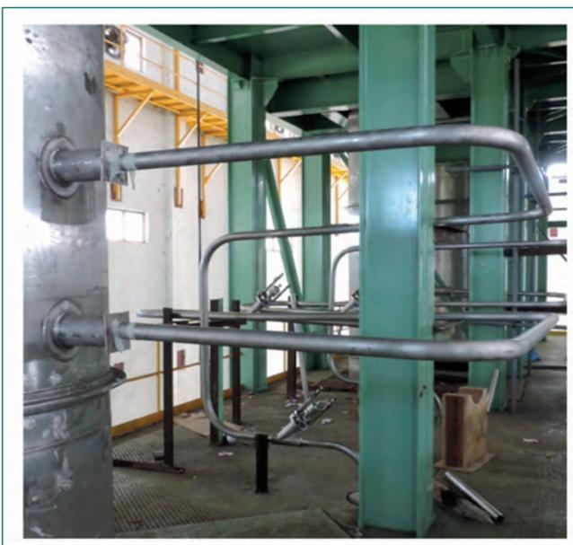
Fig. 1 Overflow and outlet pipe lines
