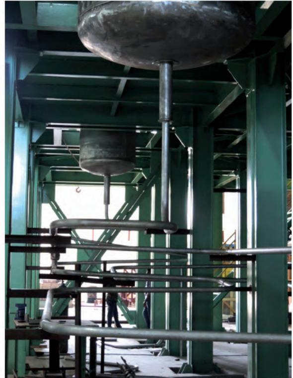
Fig. 2 Dump lines of piping system
