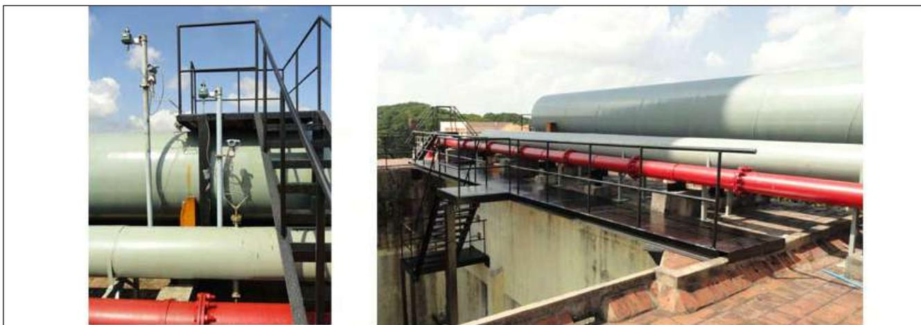
Fig.1: APT in the plant exhaust duct along with wireless adapter fitted on DP transmitter
