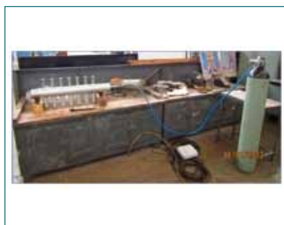
Fig.7: Nitrogen Gas Filling in fabricated sub-header
