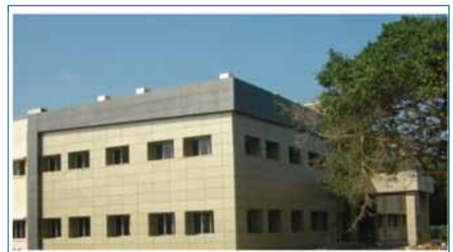
Fig 7: View of Complete Building
