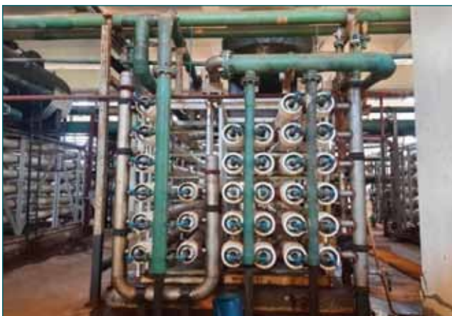
Fig. 1: Reverse Osmosis Stage 1
