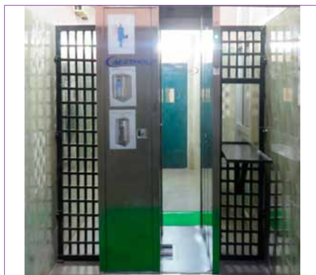
Fig.2: One way exit through portal whole body contamination monitor from active areas of FBTR
