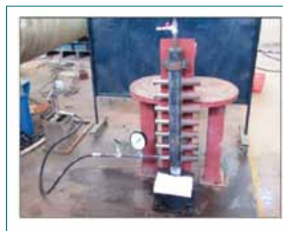
Fig.6: Hydro testing (at 250 kg/cm 2 ) of fabricated inlet water sub-header
