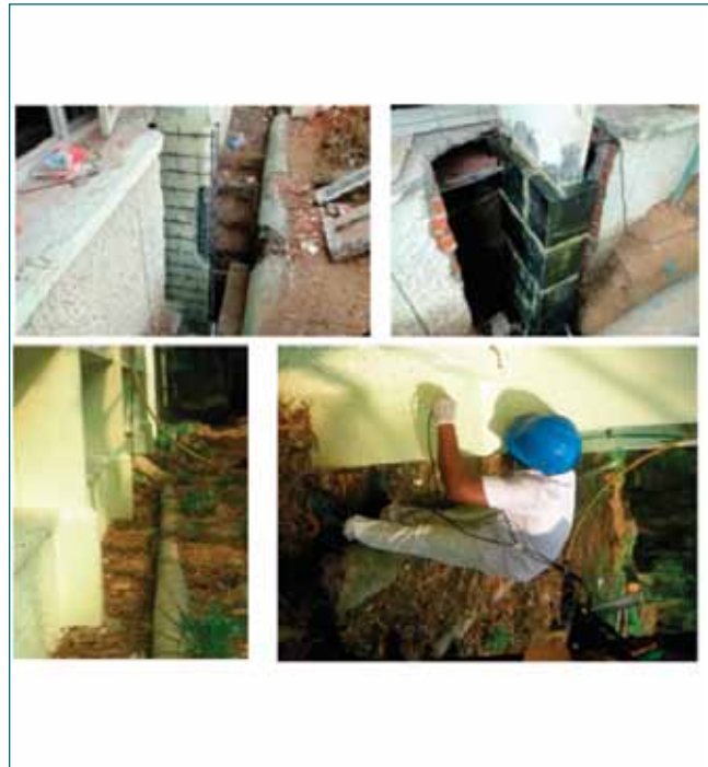
Fig. 2: Restoration of RC columns & monitoring
