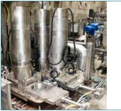
Fig. 4: Anode & cathode assembly located over HTER vessel
