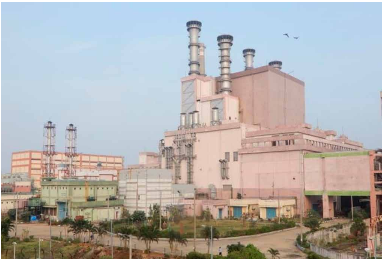
Fig. 1: Overall view of Nuclear Island and Site Assembly Shop
