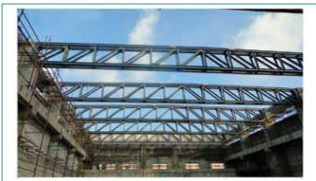
Fig 5: Truss (High bay)
