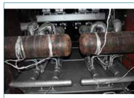
Fig.3: After replacement of Water Sub-headers
