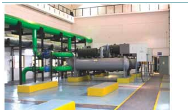
Fig. 2: CWCP-II established near IGCAR gate.
