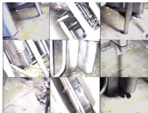
Fig. 2 : Snapshots of few equipment and vessels below the containment box obtained during the inspection campaign from the video streamline
