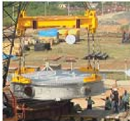
Fig. 5 : PFBR Grid Plate being unloaded at Site
