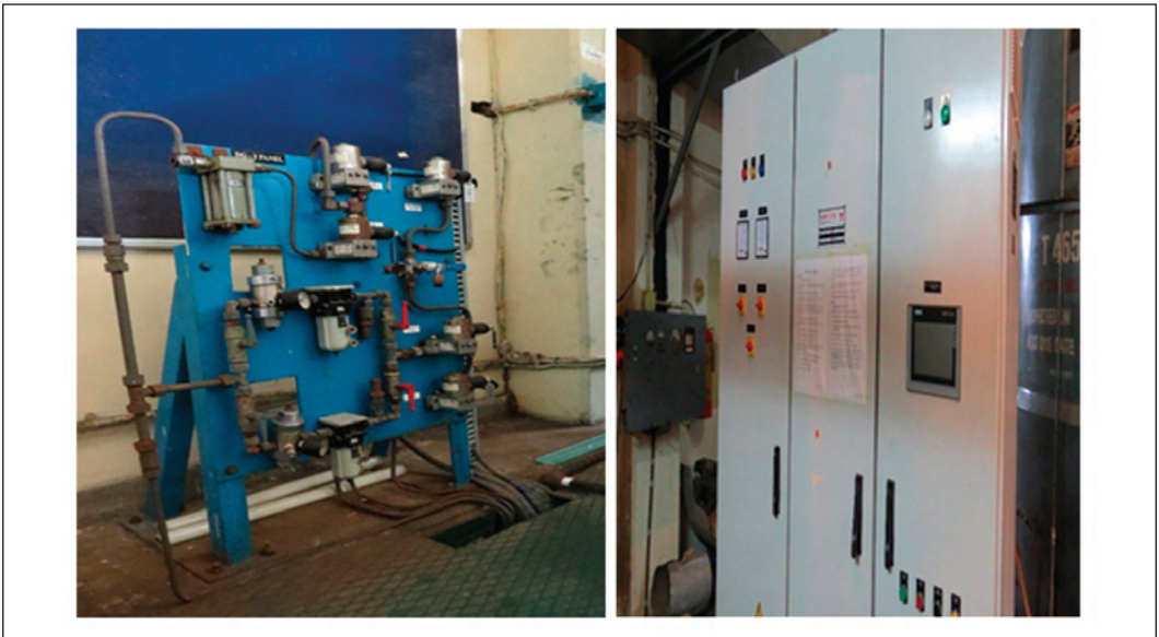
Starting air circuit DG
