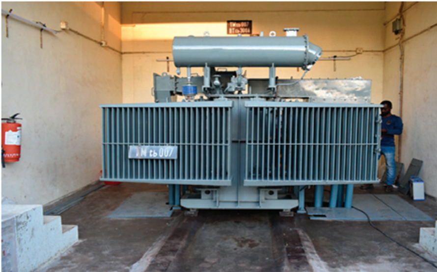
TMtb01 Transformer Installation Completed @ site
