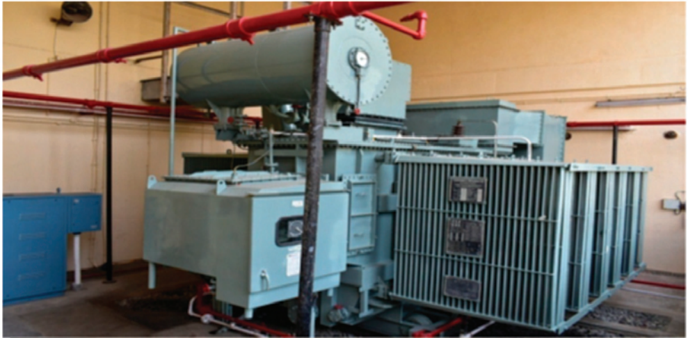
Transformer after overhauling
