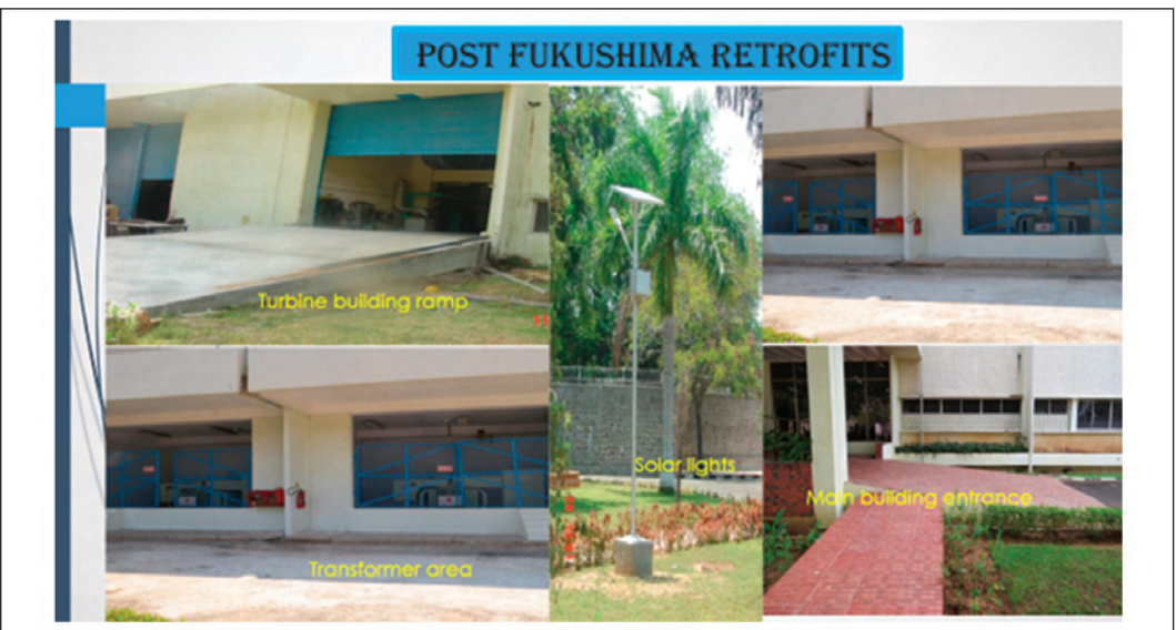
Post Fukushima Retrofits
