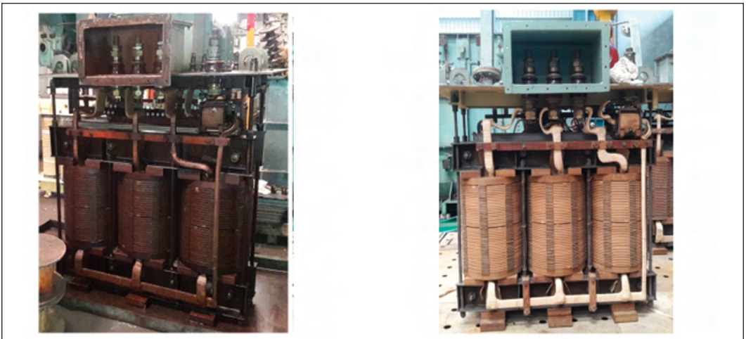
Before and after overhauling transformer TMtb07
