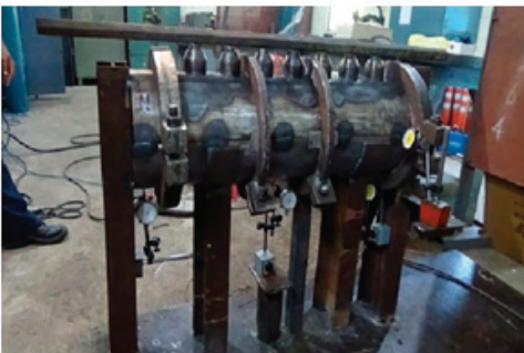
SG thermal baffles with shell root welding completed
