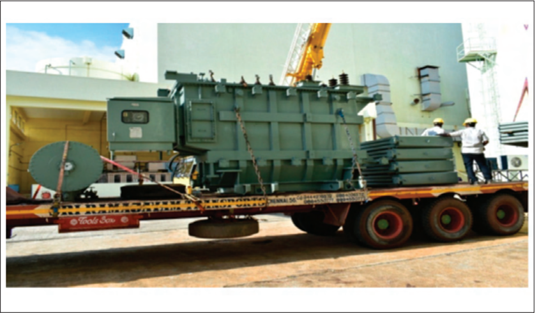
Transformer being transported to the overhauling site
