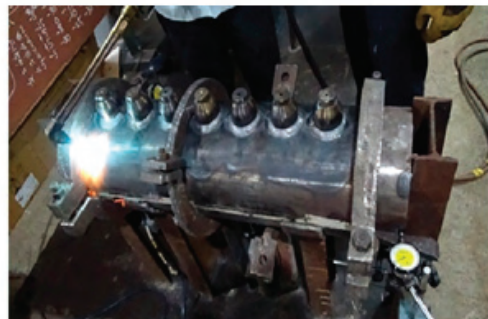
SG thermal baffles with shell final welding and heating completed
