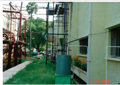
BSC leak sealing mock up set up
