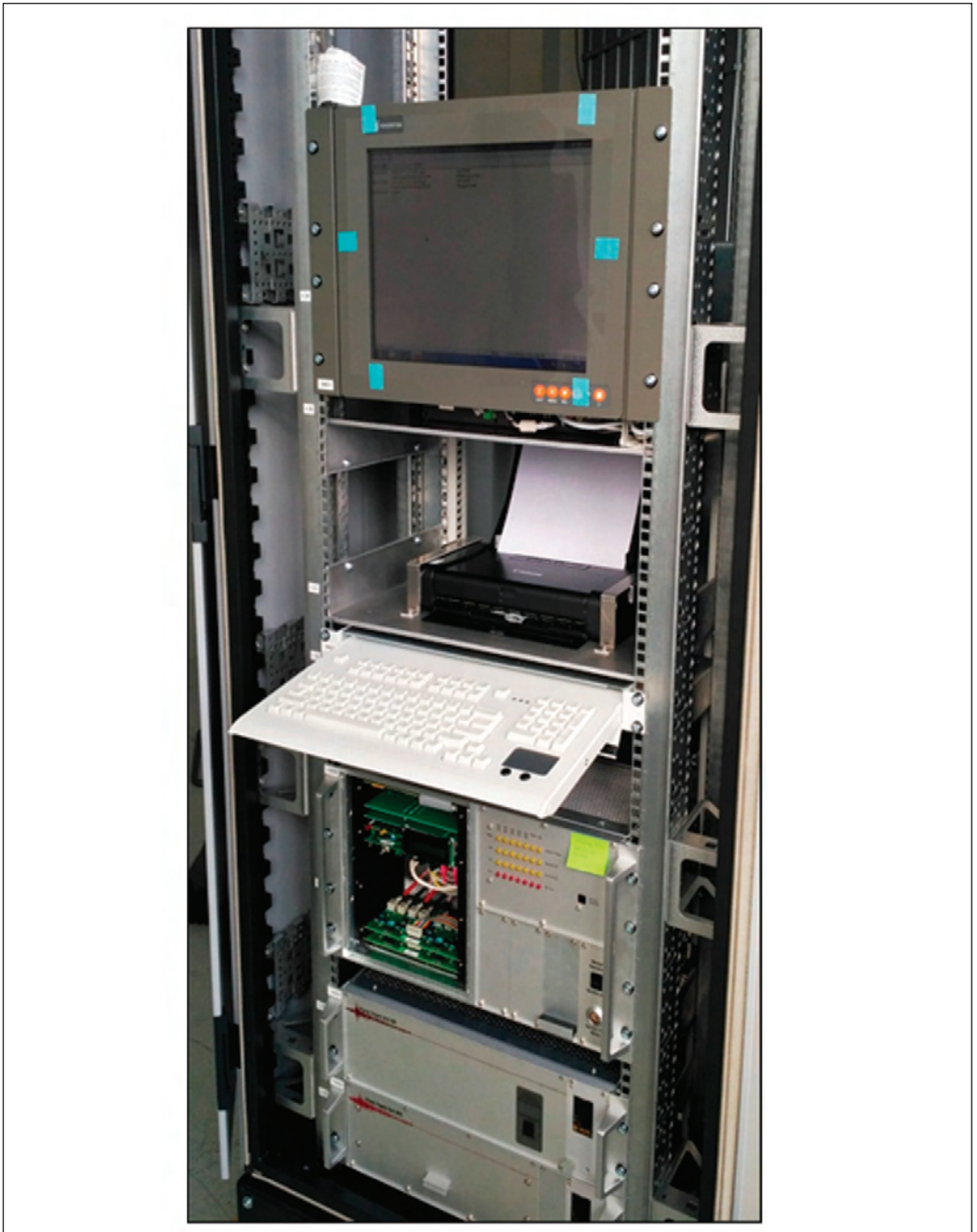
Seismic recording instrumentation in Relay room
