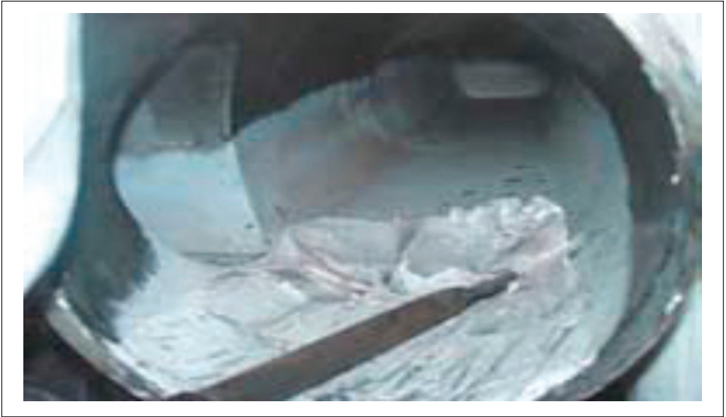
Scooping of frozen sodium from the SG inlet header
