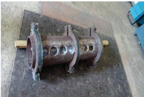
SG sodium inlet header shell prefabrication completed
