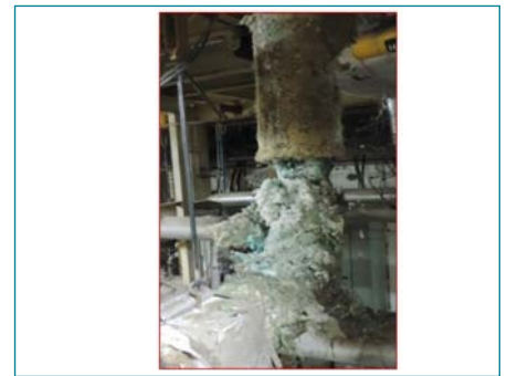
Figure 2: LCTR pipe line sodium leak
