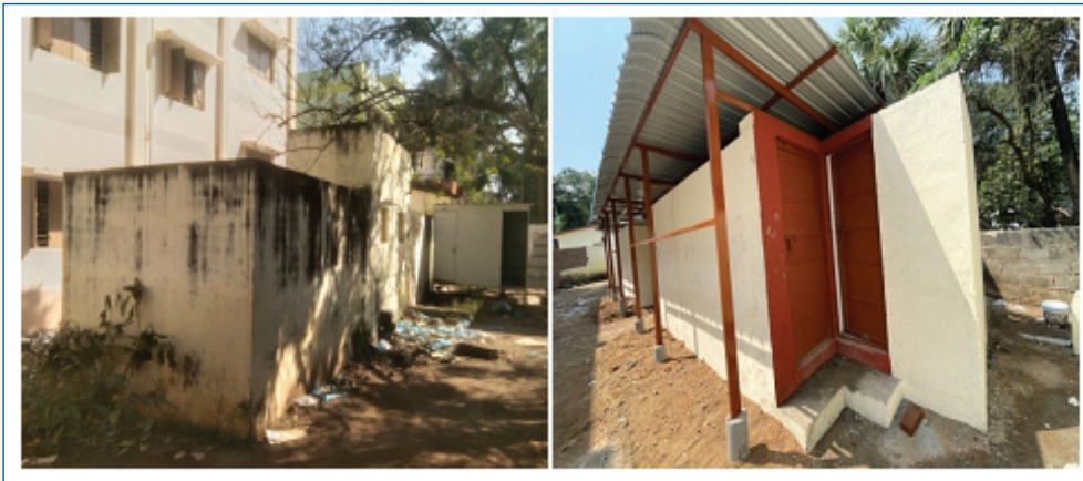
Renovated school toilets with new roof sheets
