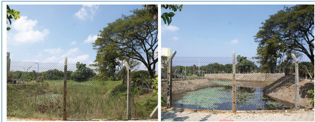
Restoration of pond near DFRP plant
