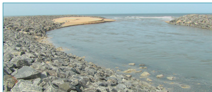
Fig. 3: Seawater outfall canal with Guided bund for PFBR
