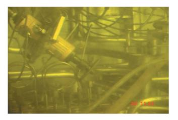
**Fig.2**Remote Cutting of Interface Airline.
