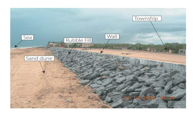
**Fig.3**Tsunami Protection Wall under Construction
