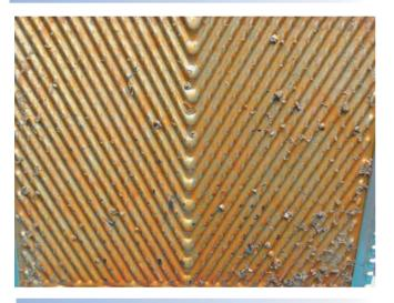
**Fig.7**A View of Silt Deposition on PHE
