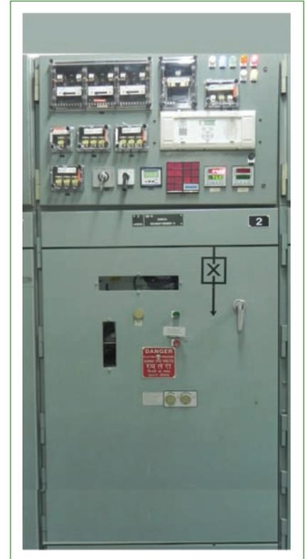
**Fig. 1** Central switching station panel with numerical relay
