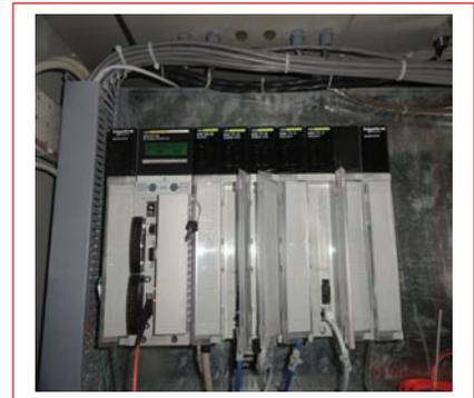
Fig.1 PLC web server module mounted in PLC rack
