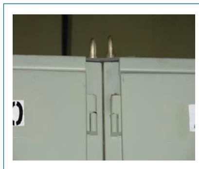
**Fig. 3** Bolting of adjacent panels to avoid seismic interactions
