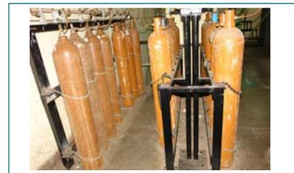
**Fig. 2** Seismic anchoring of gas cylinder banks in the plant
