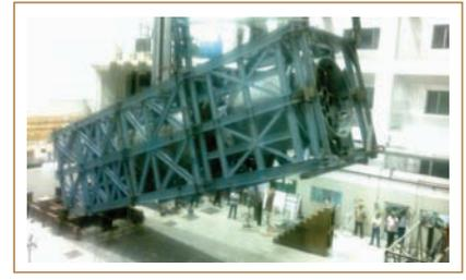
**Fig. 6** Making control plug from vertical to horizontal with handling structure
