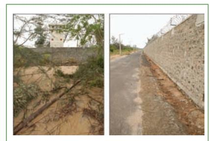
**Fig. 4** Beach erosion near Edaiyur watchtower and seepage of seawater through the IGCAR boundary wall
