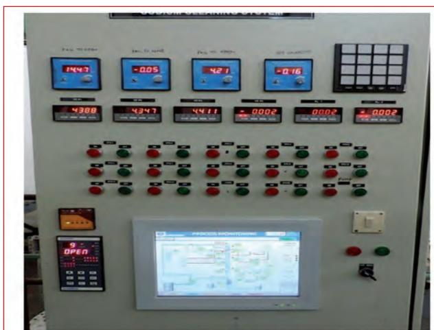
**Fig. 3** Control panel with auto/manual switches and SCADA
