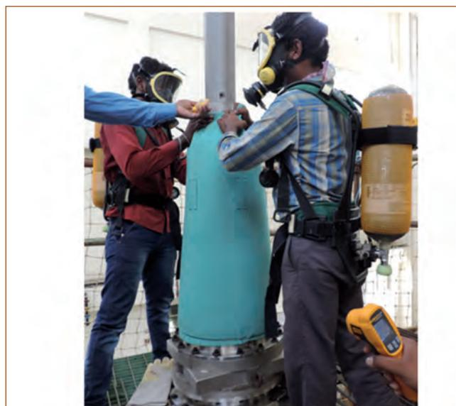
**Fig. 2** Oxygen and temperature measurements being taken and persons with SCBA
