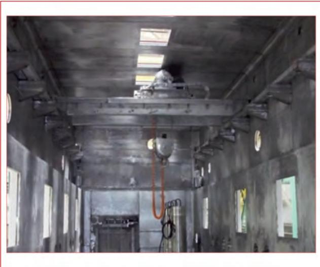
Fig. 1 In-cell crane installed in containment box
