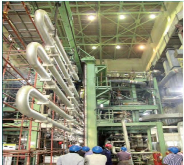
*Fig. 1 Steam generator loop*
