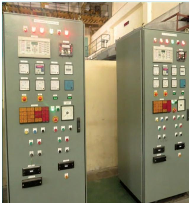
*Fig. 1 The typical state-of-the-art panels of the diesel generators of FBTR*
