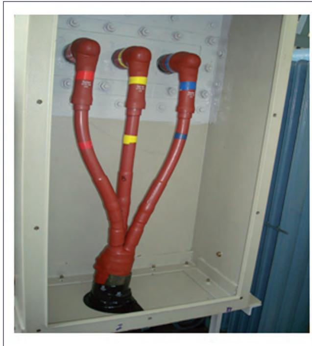
**Fig. 1** 11 kV transformer end termination - refurbished
