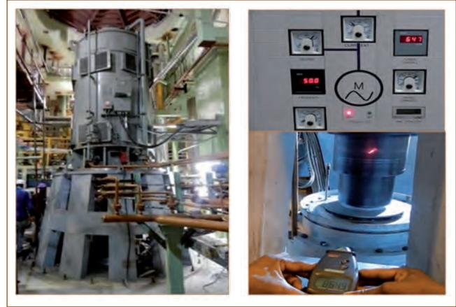
**Fig. 3** Commissioning of secondary sodium pump
