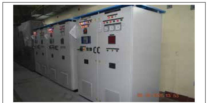
Fig. 4: New chargers installed at FBTR
