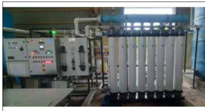
Fig.3: Reused Membranes in Service at UF Skid-2
