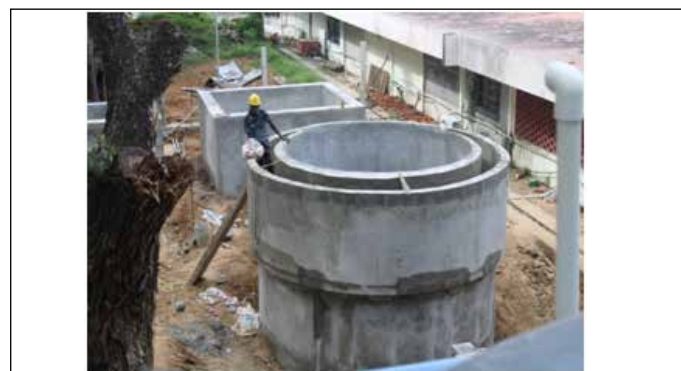
Fig.1 View of Bio gas Plant during construction
