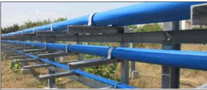
Fig. 1: 33kV Cable and OFC cable on Service corridor near UGC
