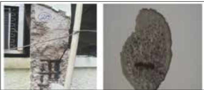
Fig.2 Distressed areas on the structural members
