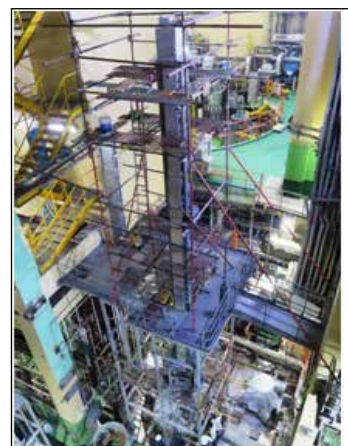
Fig. 8 Erection of PSAHF at PFBR Site
