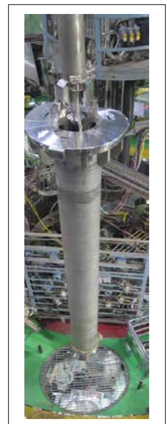
Fig. 2: TP Lowering through IVTP access port
