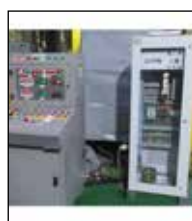
Fig. 2: Local Control Panel & VFD Panel of PSAHF
