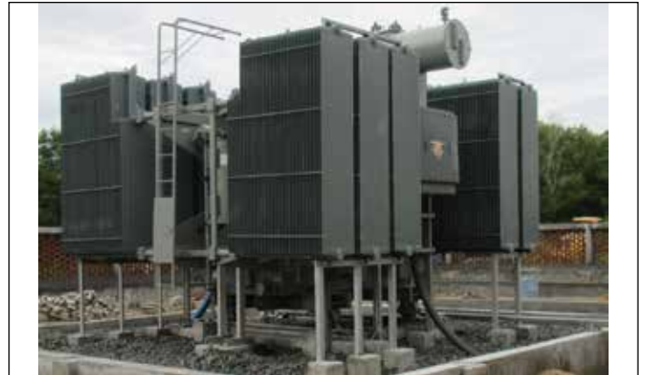
Fig. 3: 33 kV transformer and associated HT panel connections at the Northern Node.
