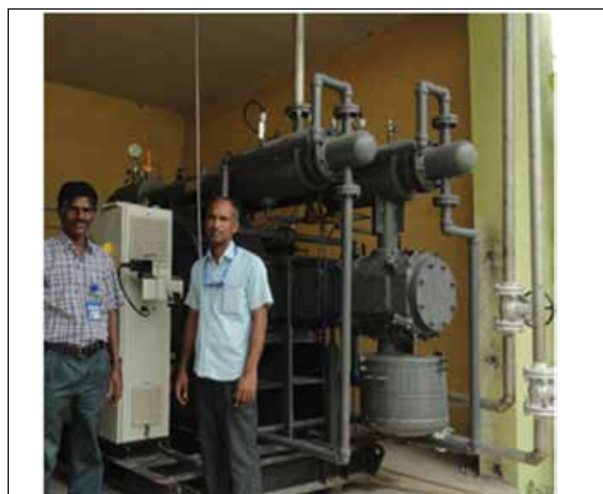
Fig.4 Two-stage 200 CFM compressor
