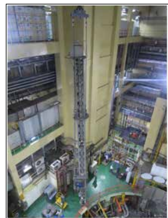
Fig. 10 Trial Movement of PFBR PSAHF within RCB
