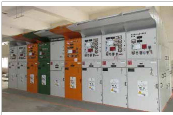
Fig. 2: 33 kV HT switchgear panels at the Northern Node
